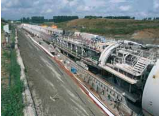
Back-up installation in front of the Section Wienerwald Tunnel
